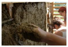
for wattle and daub it is important to use short straw. once the mixture is prepared you through the mass onto the structure and flatten it with your hand.
