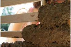
for the spaliér technique use the long straw. produce flat long patches and fold them around the wooden constrcution. afterward pastering
